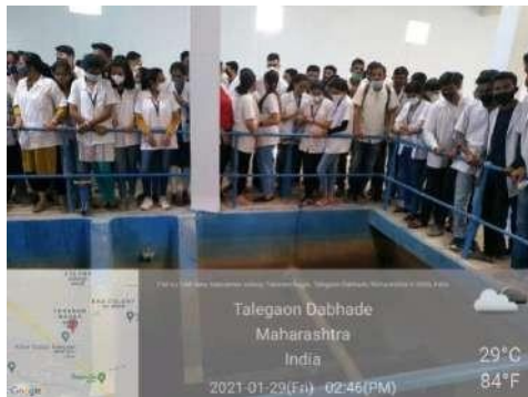
Water Purification Plant, Talegaon
